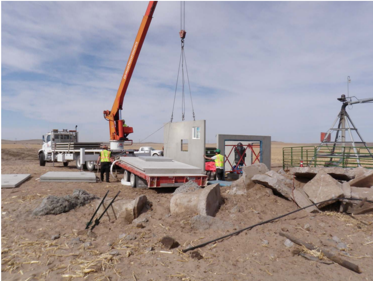
Colorado Precast installing a wall panel of well house B5.
