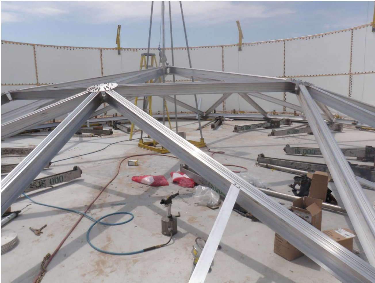
Assembly of the domed roof for the collection tank.
