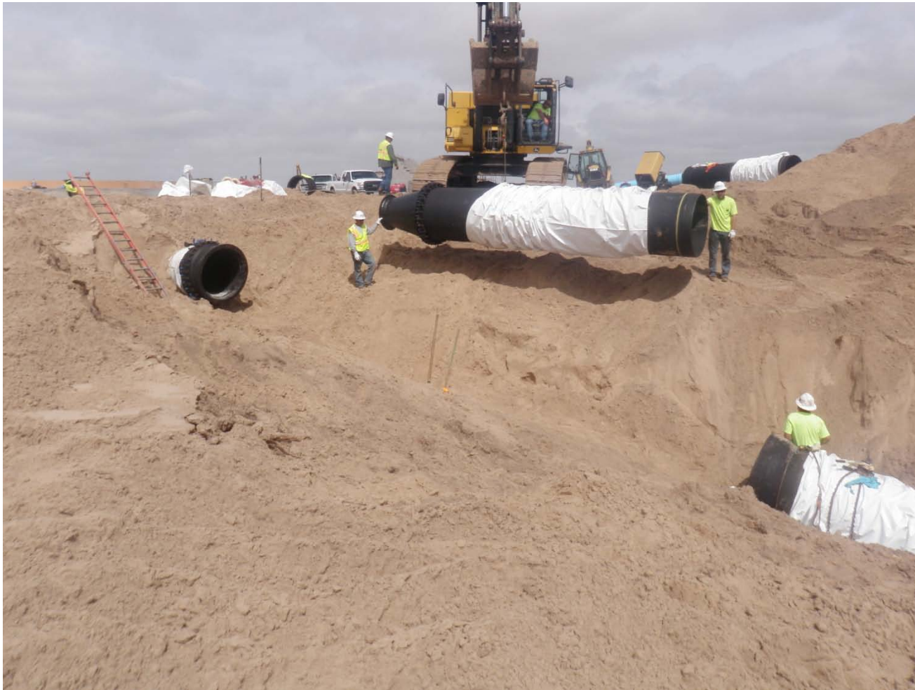
Garney placing final piece of DI pipe at collection tank site.
