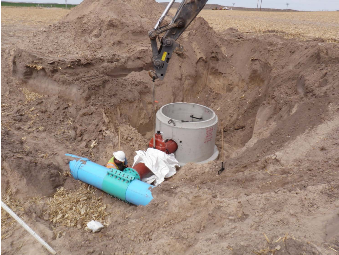
Sessions installing blowoff manhole at Station A5 44+50 on collection line.
