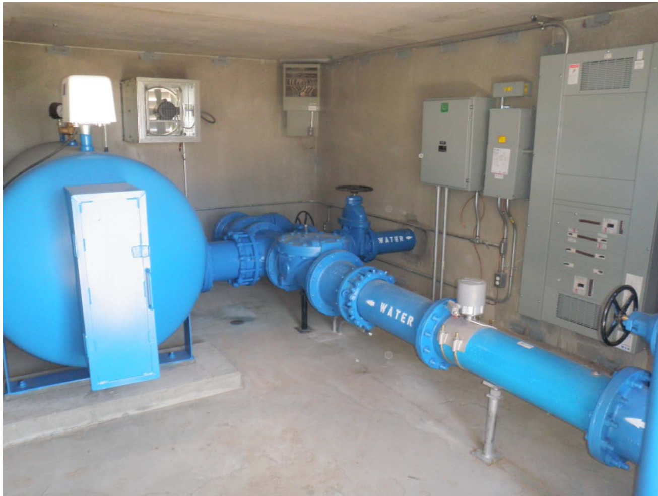
Completed interior of a well house.
