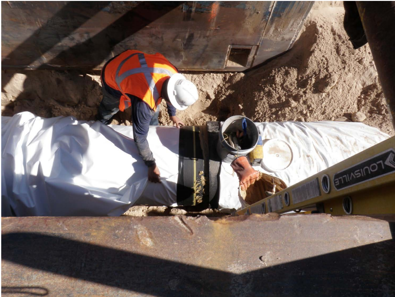
Garney installing ductile iron pipe, showing bell and spigot installation style.
