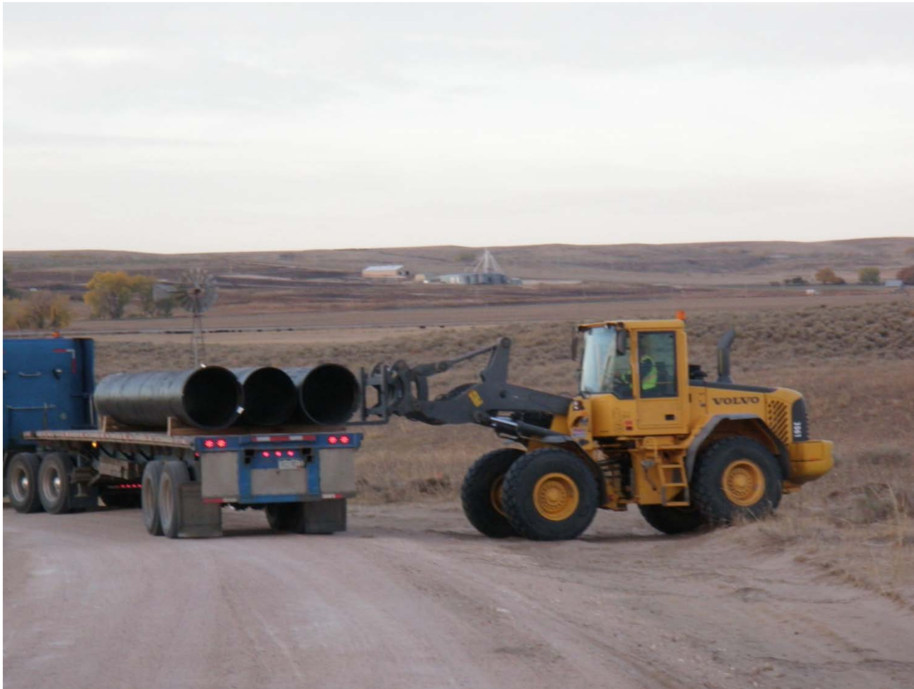
Garney unloading ductile iron pipes from delivery trailer.
