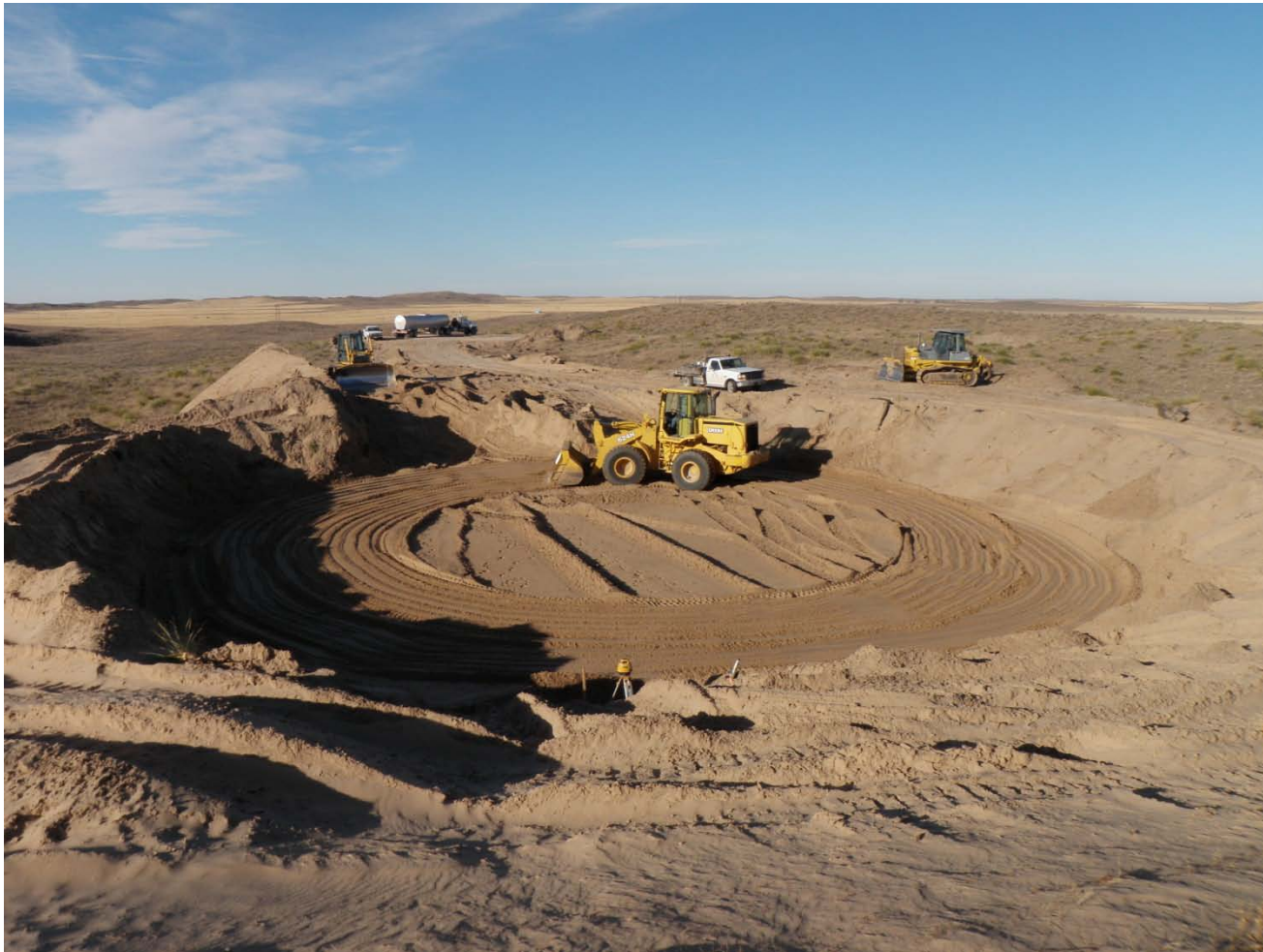
Spreading backfill under collection tank foundation before compacting lift.
