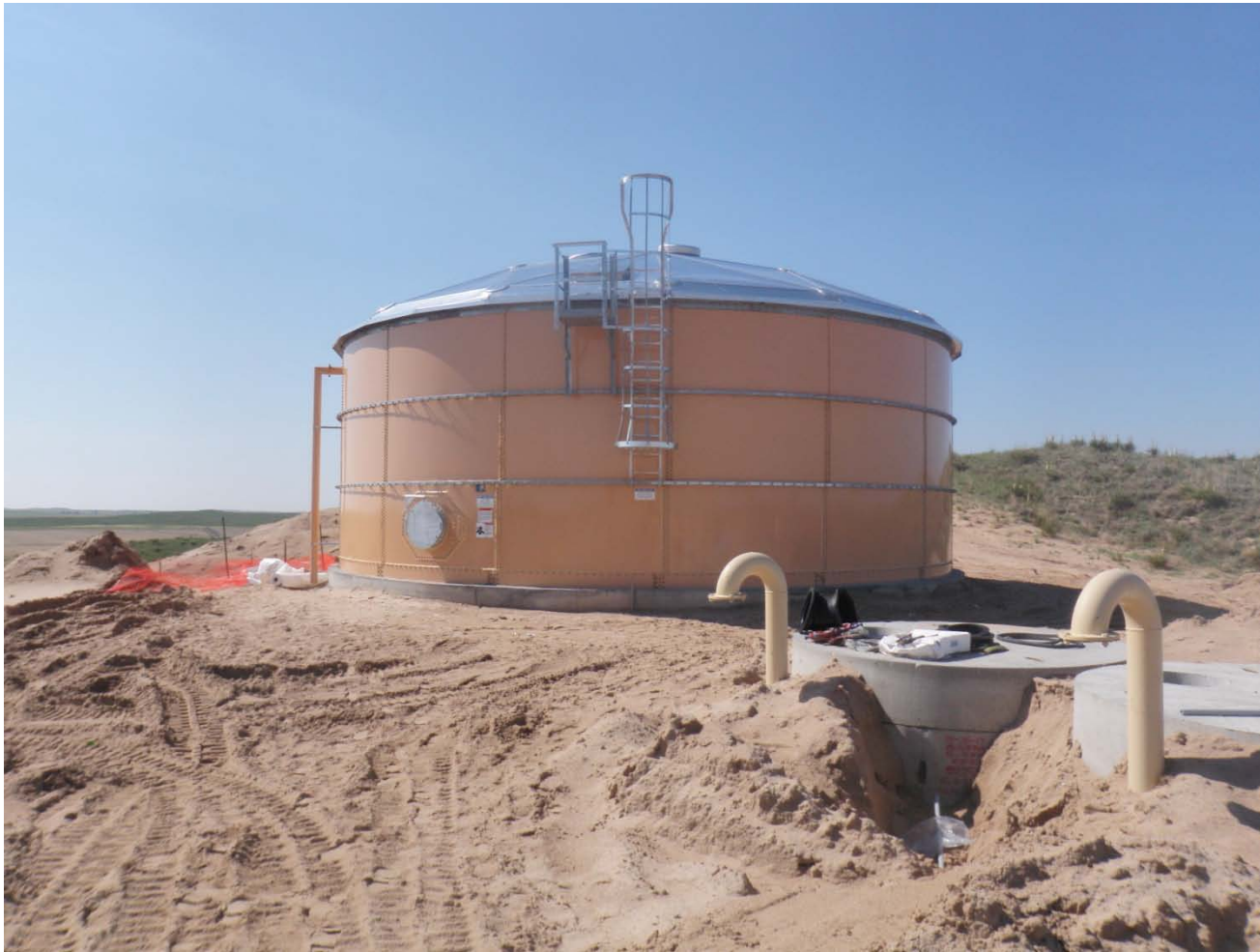
Completed collection tank.
