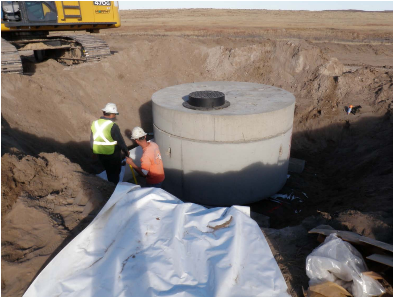
Garney installing manhole over air release at Station 45+28.
