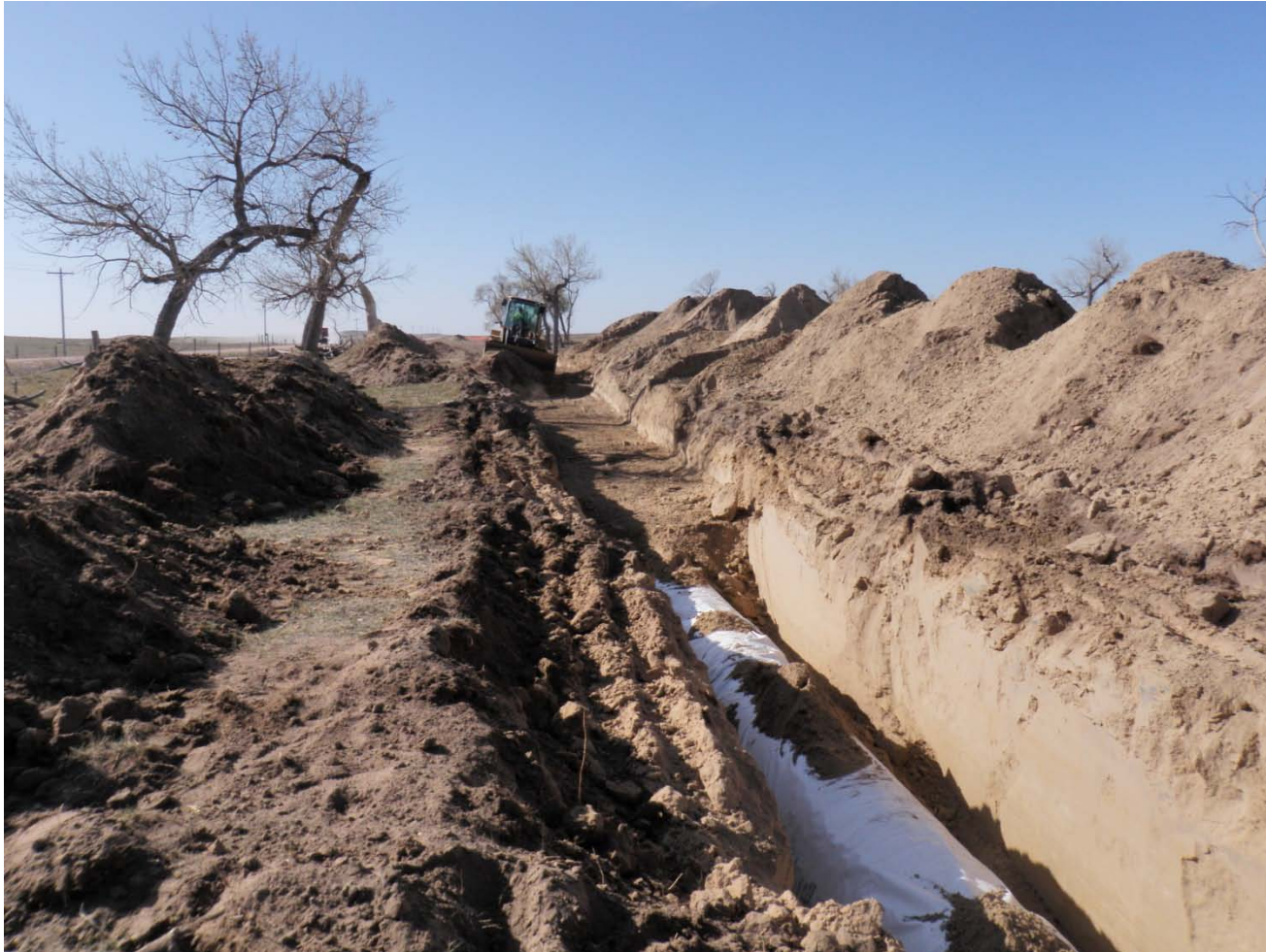
Garney backfilling trench over 42-inch ductile iron pipeline.
