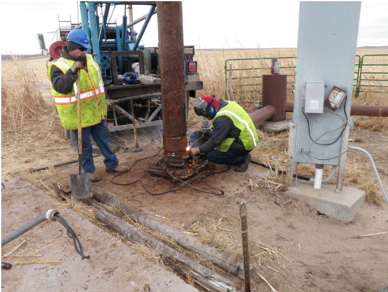
Quality Irrigation removing existing column pipe at well site A8.
