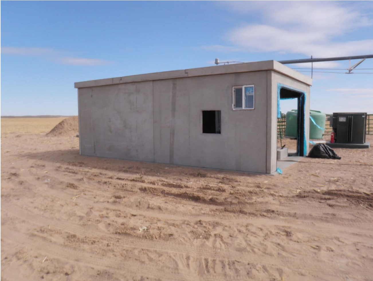
Well house A5 after Colorado Precast has completed the installation.
