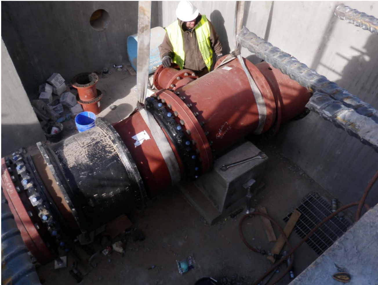
Sessions installing piping inside the outfall structure.
