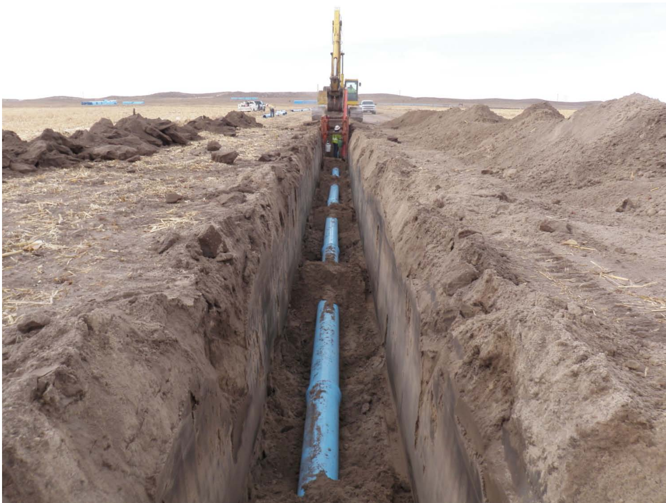
Sessions installing 12-inch PVC pipe along collection line A8, looking west.
