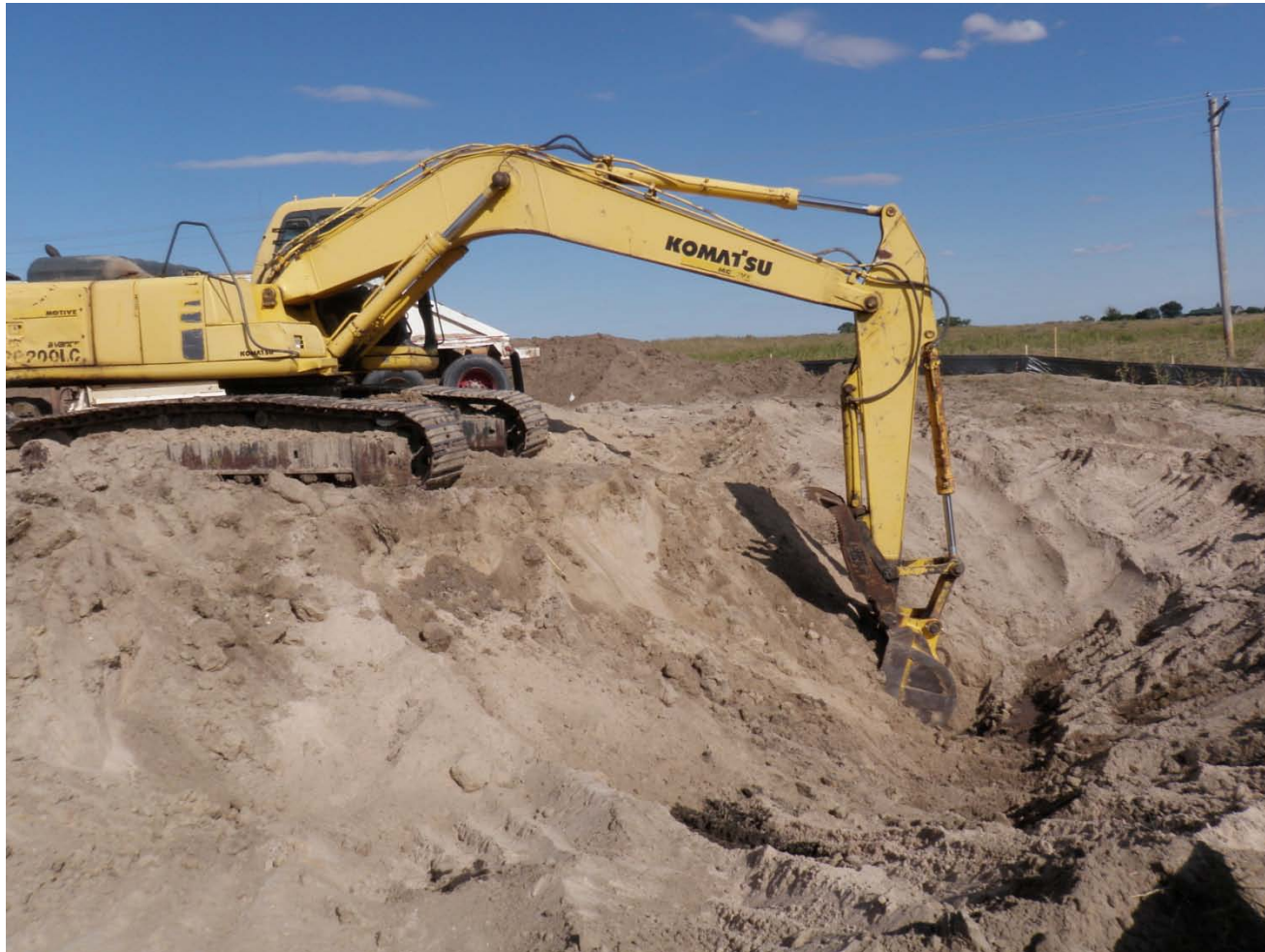
Sessions excavating discharge channel near Station 0+00.
