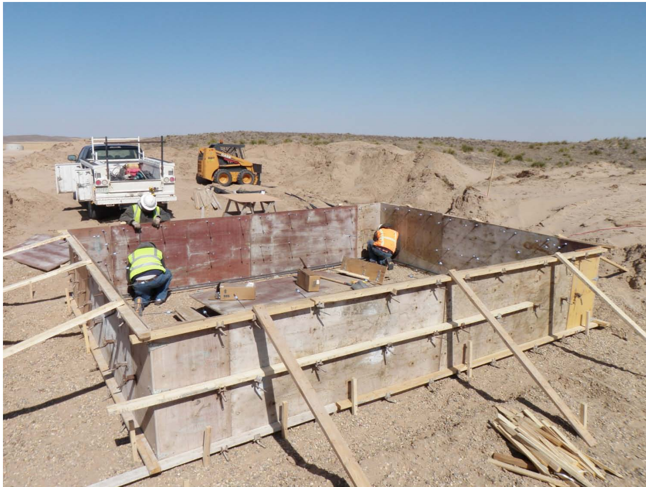
Sessions installing rebar and formwork for control building footer.
