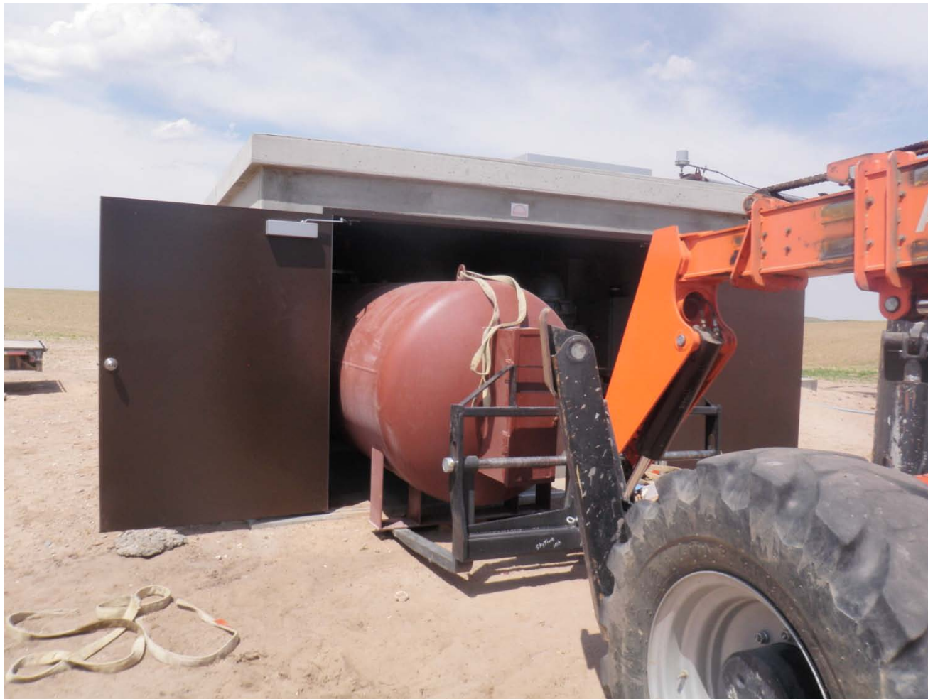
Installation of hydro-pneumatic tank in well house.
