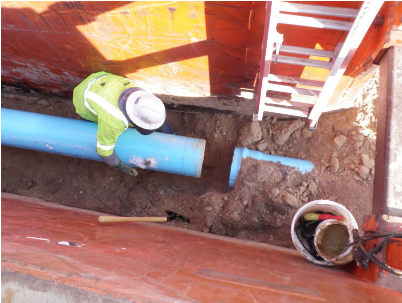
Sessions making a bell and spigot connection on a PVC well collection line.
