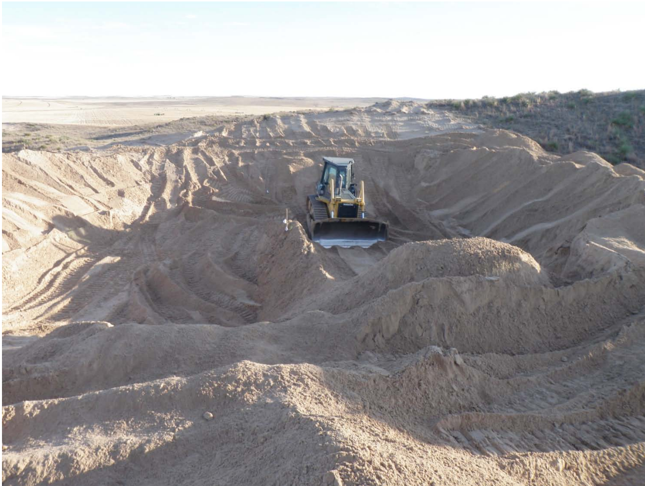
Sessions overexcavating soil underneath collection tank.
