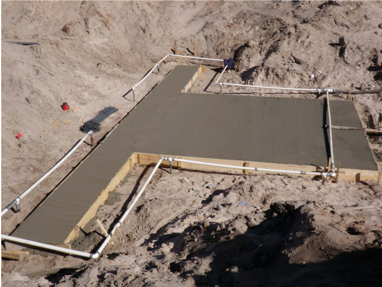
Concrete slab under Parshall flume after placement and finishing.
