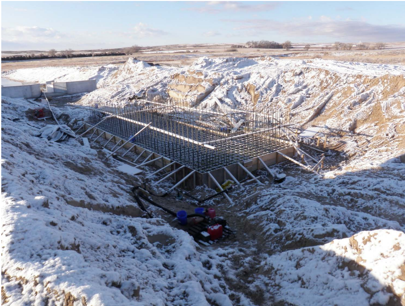
Outfall structure slab rebar mat tied and ready for concrete placement.
