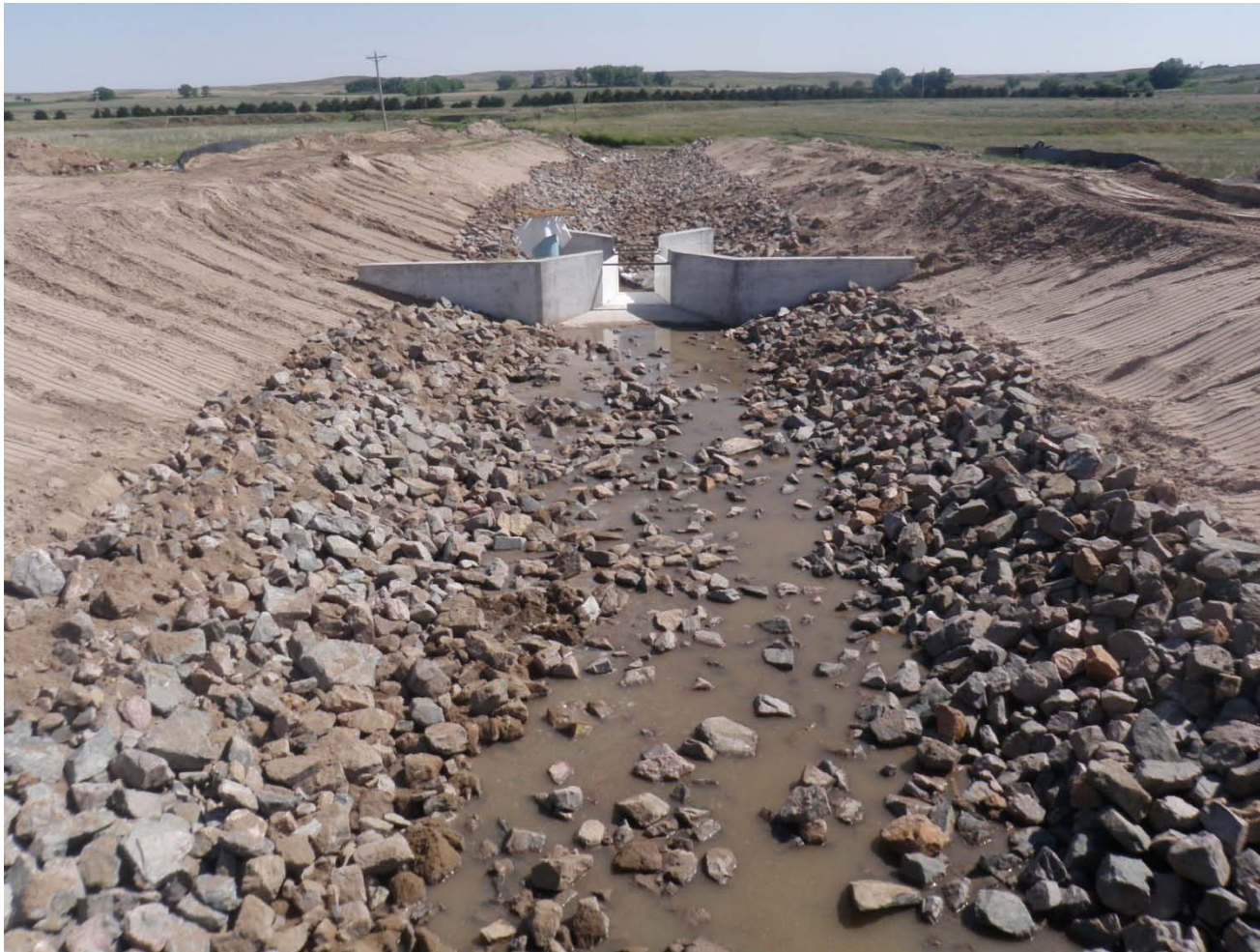
Rip rap lined outfall channel.
