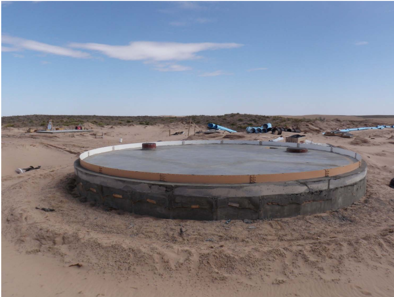
Collection tank and control building after placing both concrete slabs.
