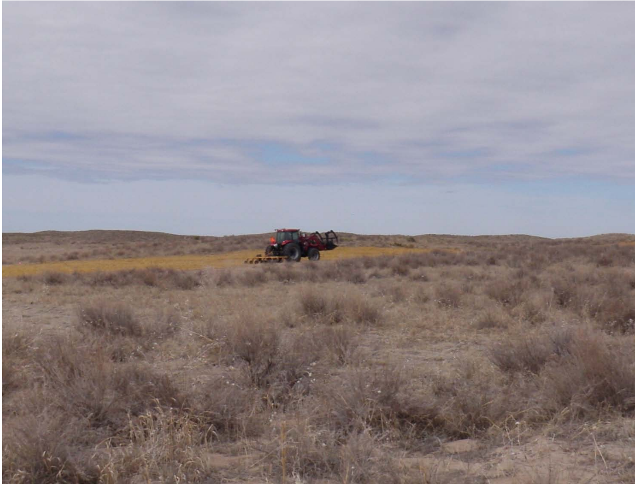
Shaw Equipment performing site reclamation within temporary easement.
