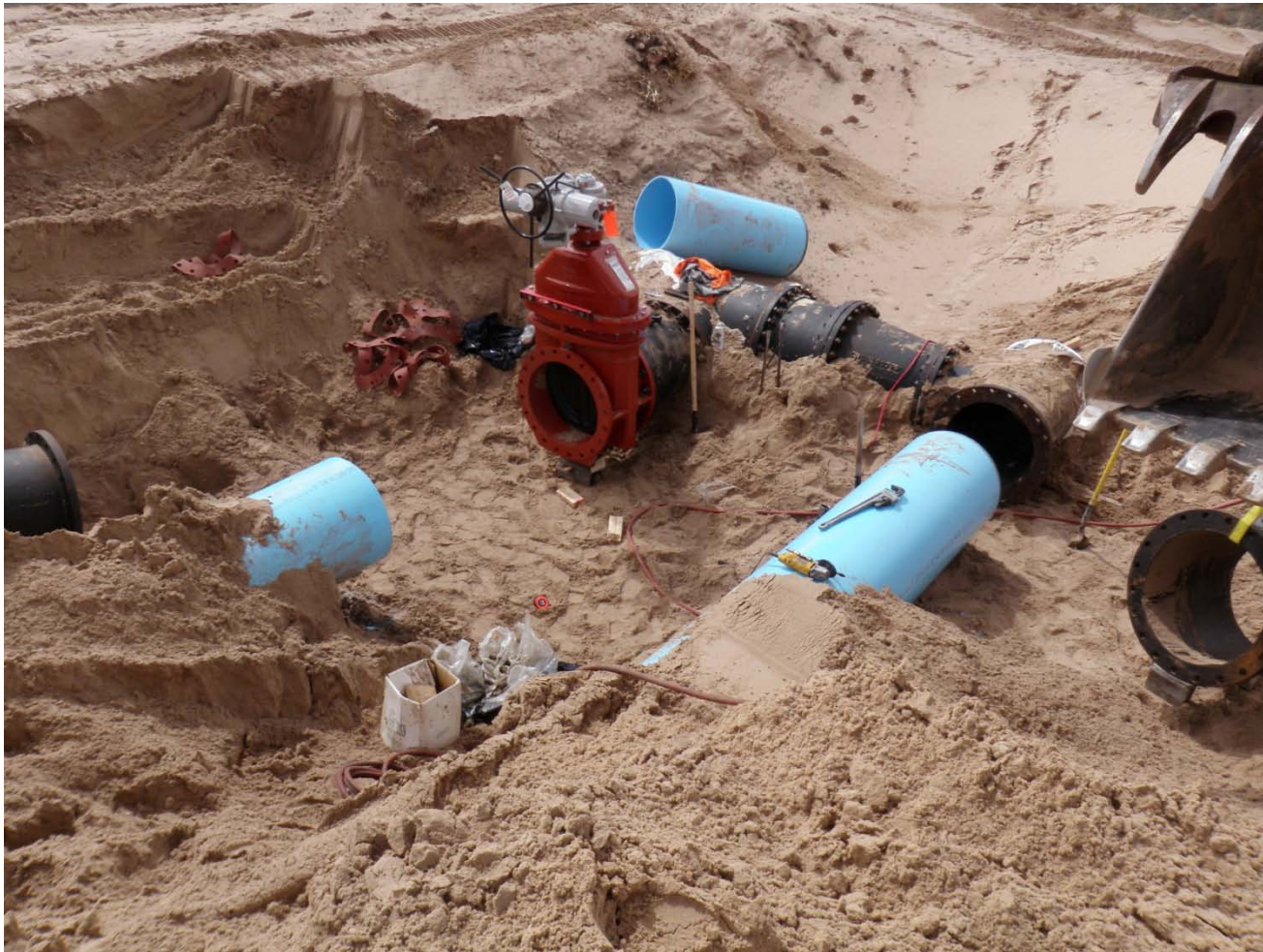
Pipe and gate valve installation at well field manifold.
