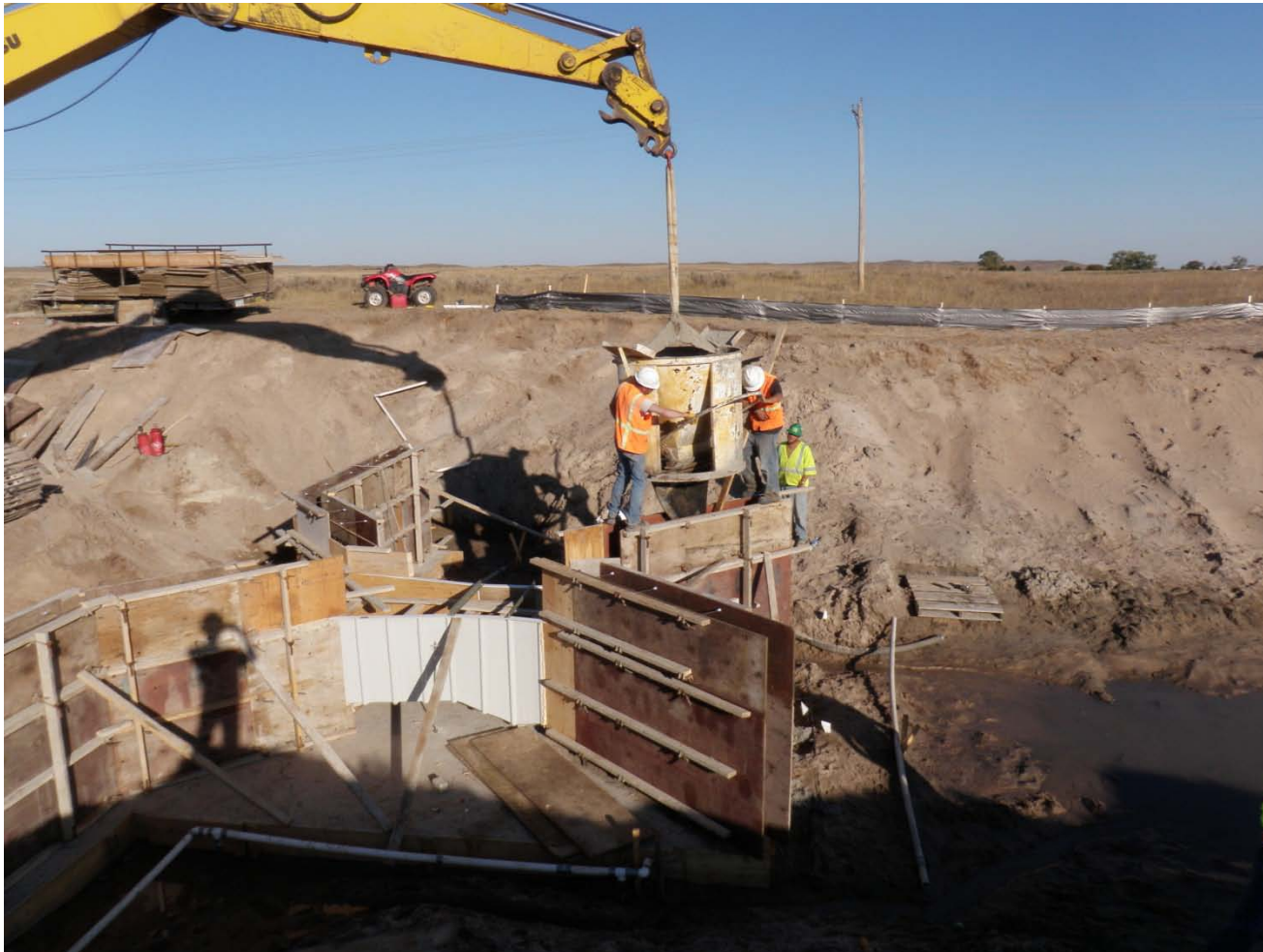
Sessions placing concrete with hopper bucket in Parshall flume wing walls.
