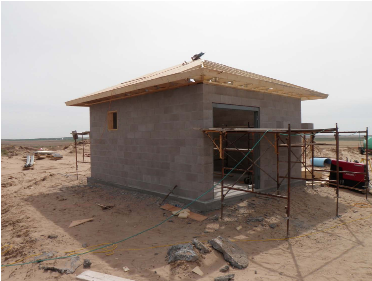
Construction of the masonry control building at the tank site.
