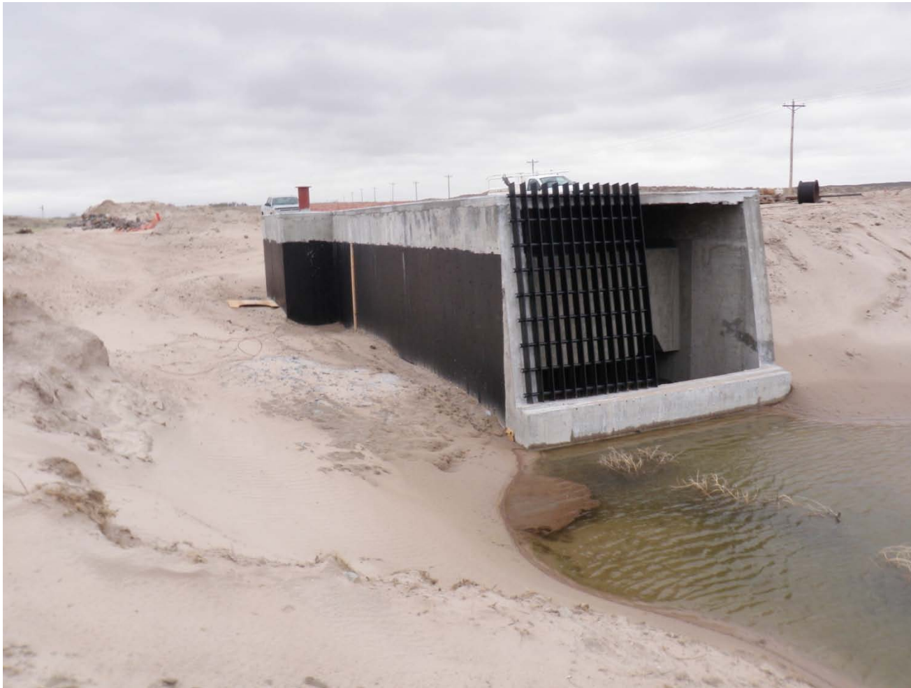
Outfall structure after roof placement with trashrack partially installed.
