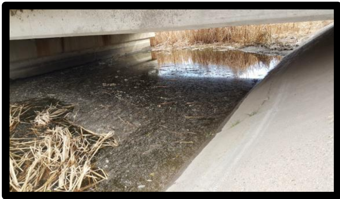
Photo 4: Highway 385 Bridge – silt and cattails have reduced clearance from 8+ feet to 3-4 feet
